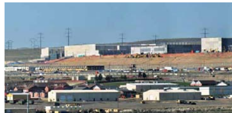
You can always retrieve that lost e-mail: The Utah Data Center, also known as the Intelligence Community Comprehensive National Cybersecurity Initiative Data Center, under construction near Bluffdale, Utah. PHOTO: SWILSONMC
