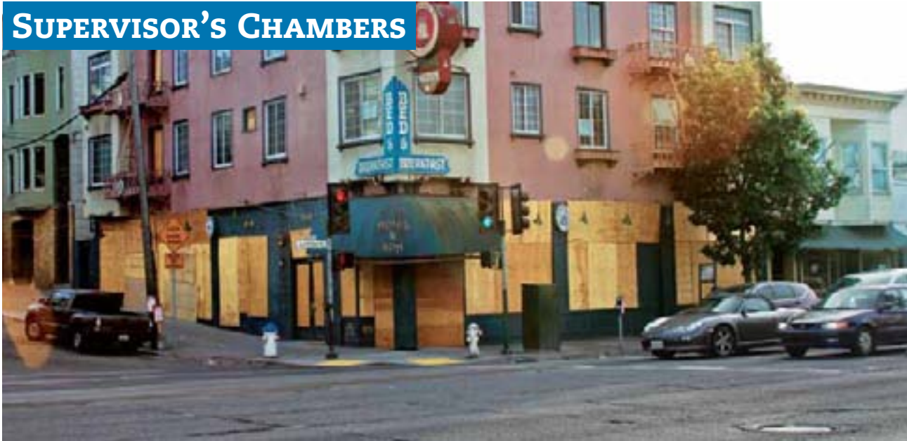
Poor road conditions and derelict buildings are among the issues plaguing Lombard Street PHOTO: STEVEN FROMTLING
