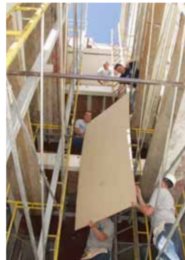
City leaders are seeking innovative ways to stimulate affordable housing development; they are not talking about bringing in the military, but U.S. sailors did pitch in for this Habitat for Humanity affordable housing project in the city. PHOTO: U.S. NAVY / AVIATION ELECTRONICS TECHNICIAN AIRMANDRA GOMES
