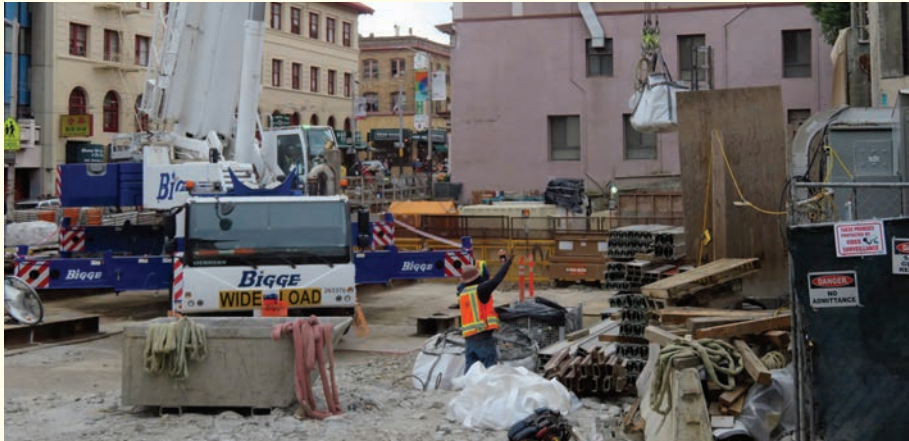
Construction of the Chinatown station in April 2019; the station will now be named after the late activist and political power broker Rose Pak. PHOTO: PI.14159265
