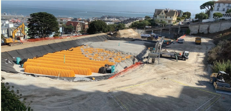
The water storage system was built in October on the site of the new Francisco Park. PHOTO: NAOMI ROSE
